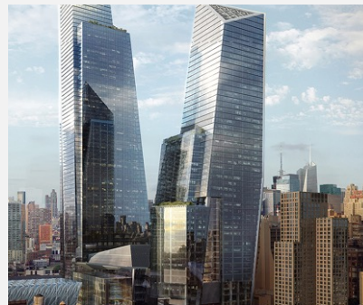
10 HUDSON YARDS New York City, NY 99% Occupancy
